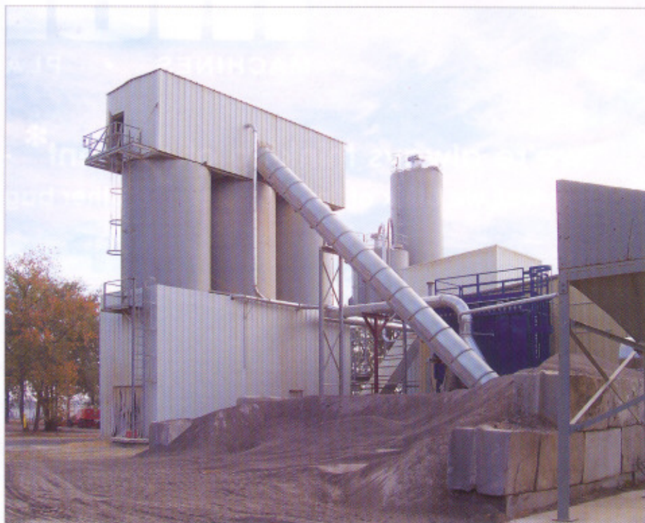
Contract haulers deliver flyash and bottom ash from coal fired power plants to Charah's manufacturing plant in Emporia, Virginia, USA.
