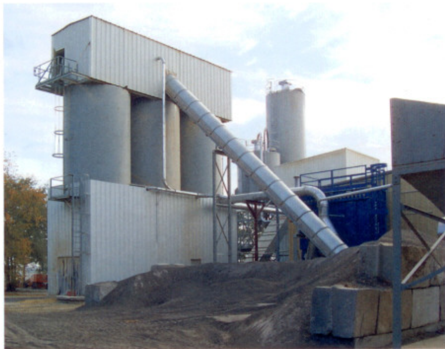
The processing plant mixes lightweight bottom ash with sand, gravel, fly ash, and cement to produce and package up to 20 different cement products.
