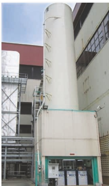
Lime Silo and Dosing System with Multiple Loss in Weight conveyors as part of an energy from waste Flue Gas Treatment Plant in Singapore.
